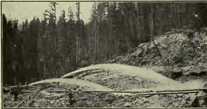
FIG. 289. — These powerful streams of water wash the gravel away, and the gold collects in the bottom of troughs, or sluices. This is called hydraulic mining.
